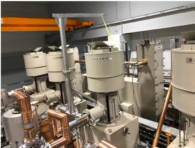
4 RF units of 200 kW/200 MHz
