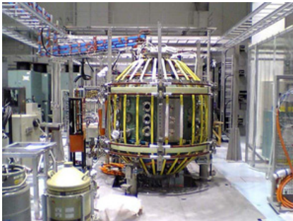
図 6.2.5: TST-2 at Kashiwa Campus.
